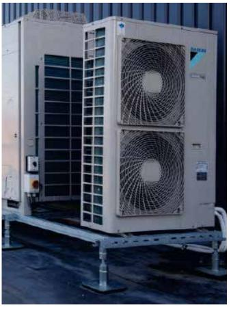
Air source heat pumps can be located on the topmost rooftops.
