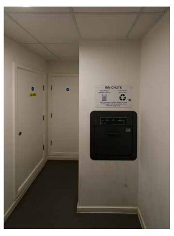
An ineffective waste chute. It is not located in a special room, signage is unclear, the area lacks ventilation and the surrounding area would be easily damaged if waste was left on the floor.
